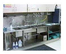
Sink manifold, lumen flush, and spray gun
